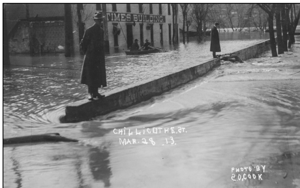
Old Portsmouth Times Building, Chillicothe St. at Front St., March 1913 flood ( Local History Digital Collection, Scioto County Public Library ). The two men are standing on the eastern end-section of Portsmouth's first floodwall, which was built to a height of 61 feet – but did it actually protect Portsmouth against a 61-foot flood?
